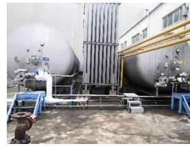
On-site equipment for renovation of regeneration gas source in hydrogen station
